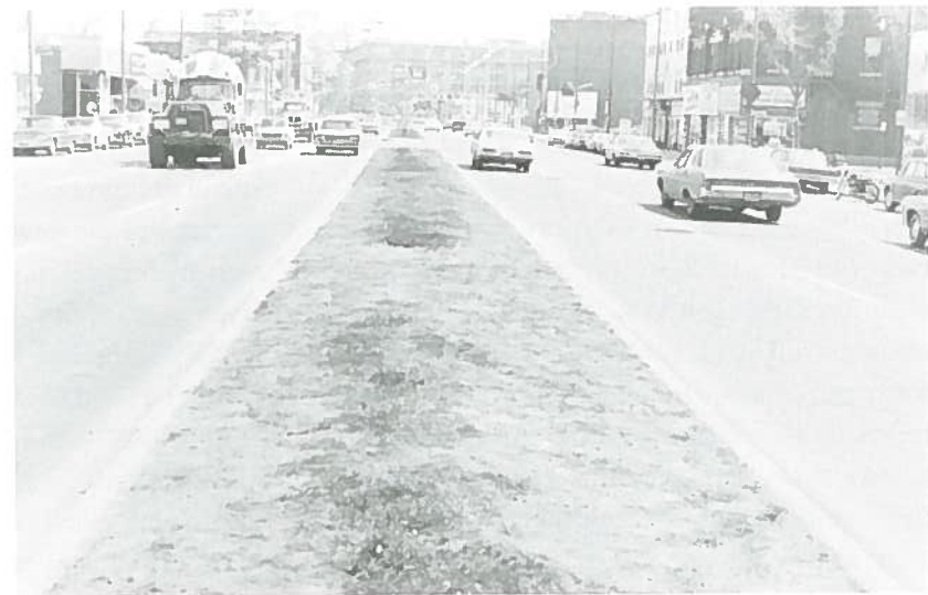
The Portage Avenue median in spring, showing damage to the grass from salt and grit-laden snow, 1971. WPRD.
