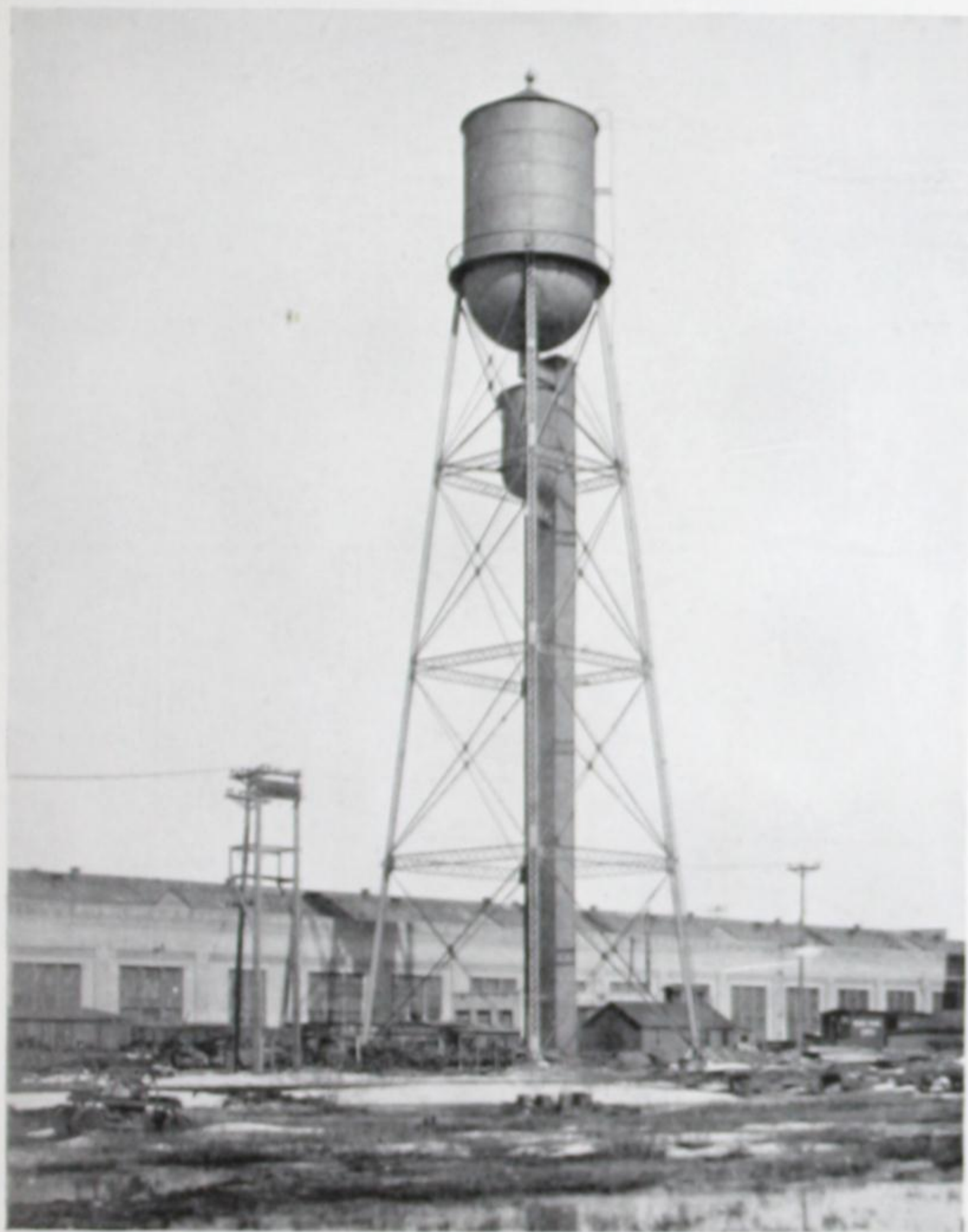
No. 93 —Elevated Water Tank at Transeona, Man., Capacity 125,000 Gallons, with Suspended Drinking-Water Tank.
