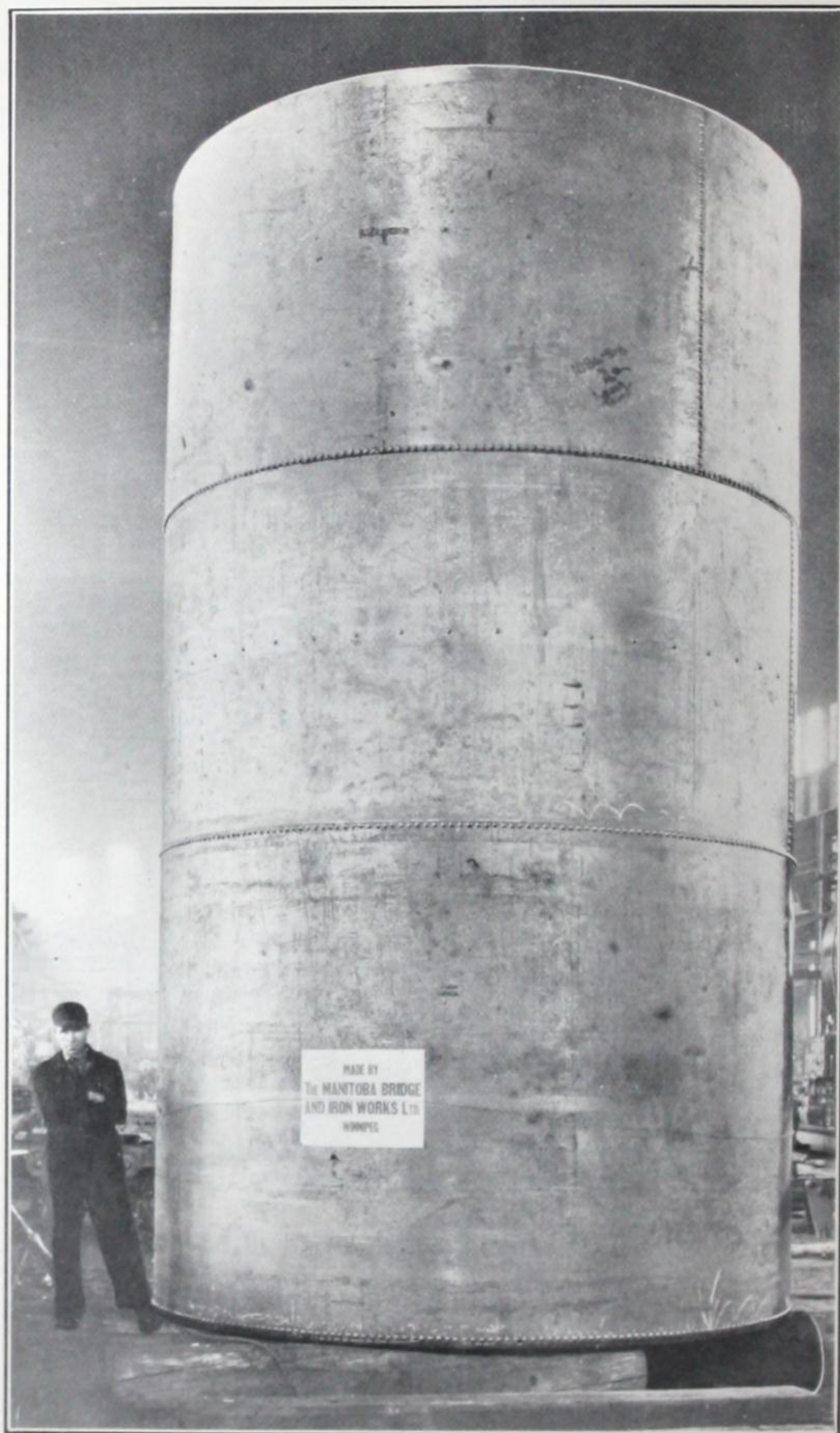
No. 94—Vertical Storage Tank with Rivetted Seams
