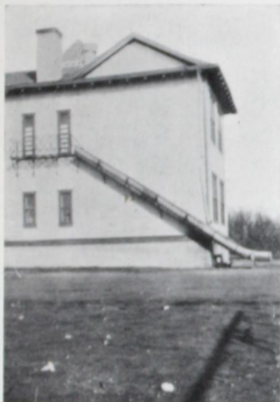
No. 52—Chute Fire Escape
