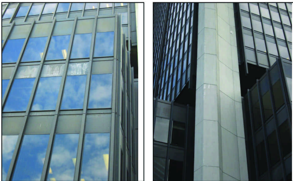
Bottom left and right La Bourse, anodized aluminum finish failure on the north side of the building.
