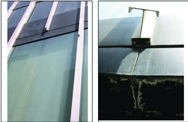
Middle left to right; Telus building damage and finish failure on the west side of the building;
